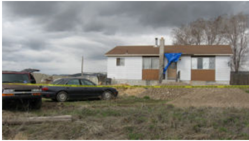
Three people were found shot to death in this home, site of suspected dogfighting and drug operations
